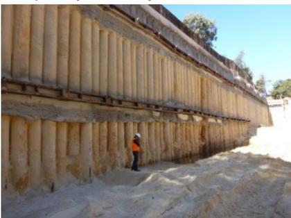
plant. EI supervised the installation of a contiguous shoring pile retention system and foundation piles for the development.
